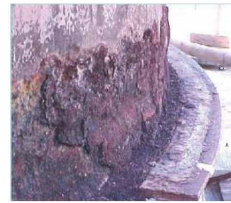
CUI at an Insulation Support Ring
